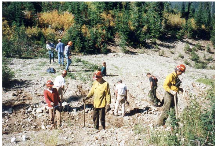
Workers hand-plant native vegetation to restore a stream crossing during road decommissioning on the Flathead National Forest. Keith Hammer photo.
