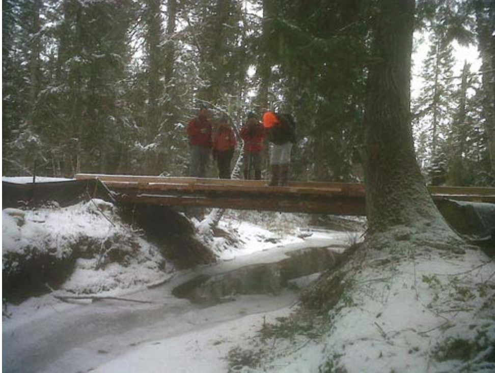
A new bridge constructed this fall over Noisy Creek.
