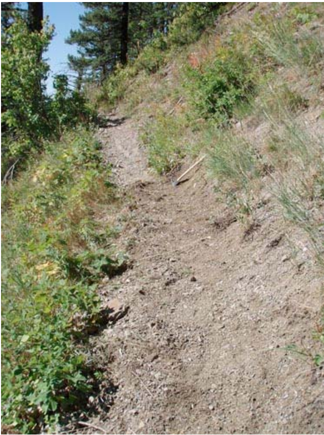
Some trail repair along the way!
