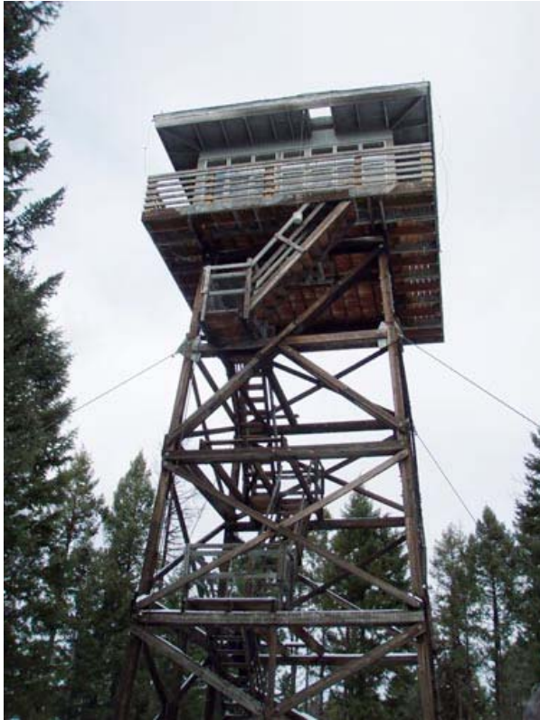
The stairs are accessible, though the observation deck is locked.
